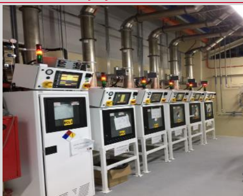
Exhibit 2a: UHP delivery system – Gas cabinet
