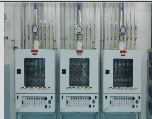
Exhibit 2b: UHP delivery system – Valve panel
